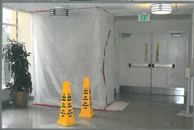
1st Floor Corridor Project
